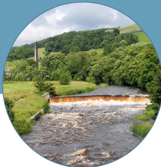
Weir impounding structure
