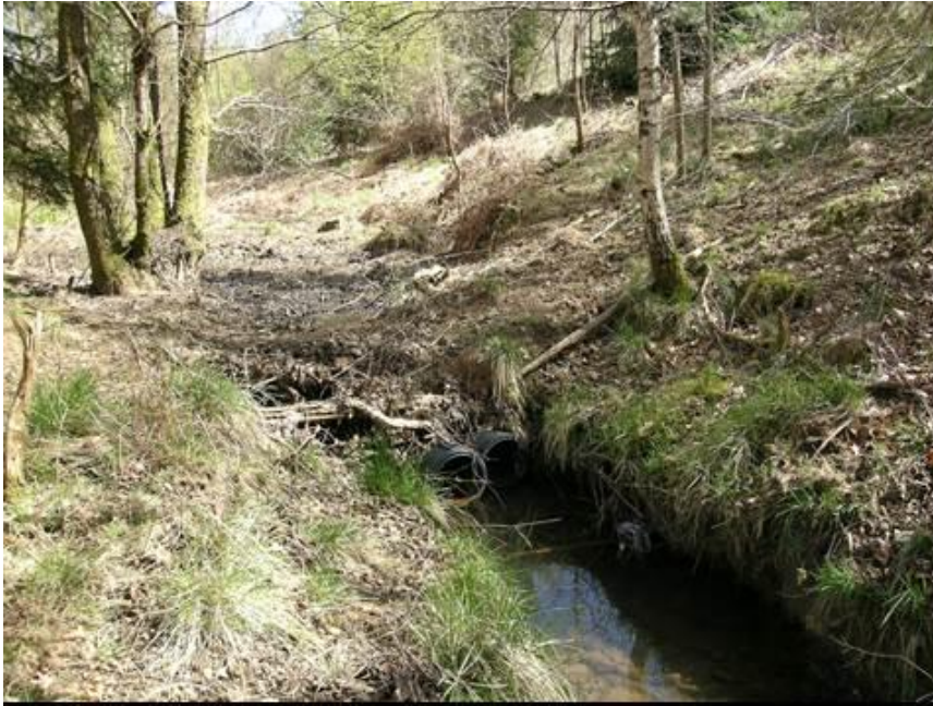
Figure 2.4 A culvert near the top of the ghyll.
