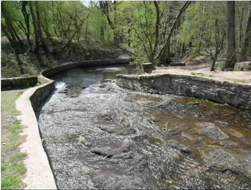
Figure 2.6 Rock spillway at the impoundment for the middle pond.
