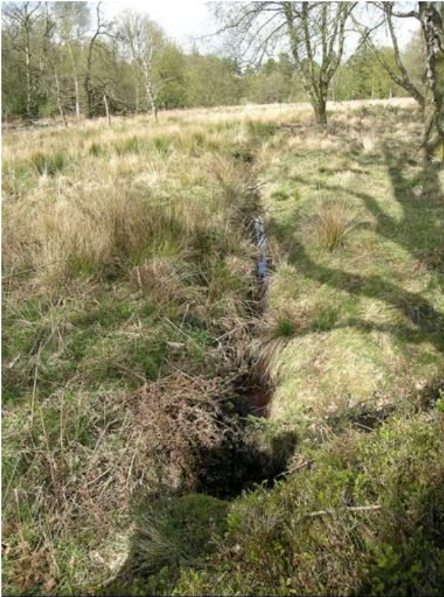
Figure 1.15 Ditch draining the central part of the mire, looking up the valley from the inclosure wall.
