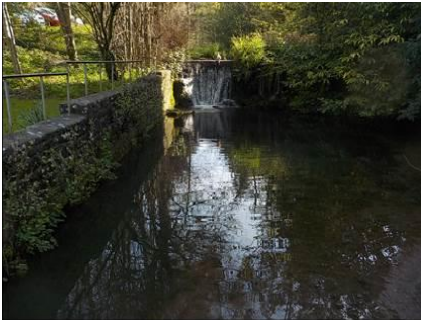
Figure 3.15 Weir on Mork Brook in the grounds of an old Country House.
