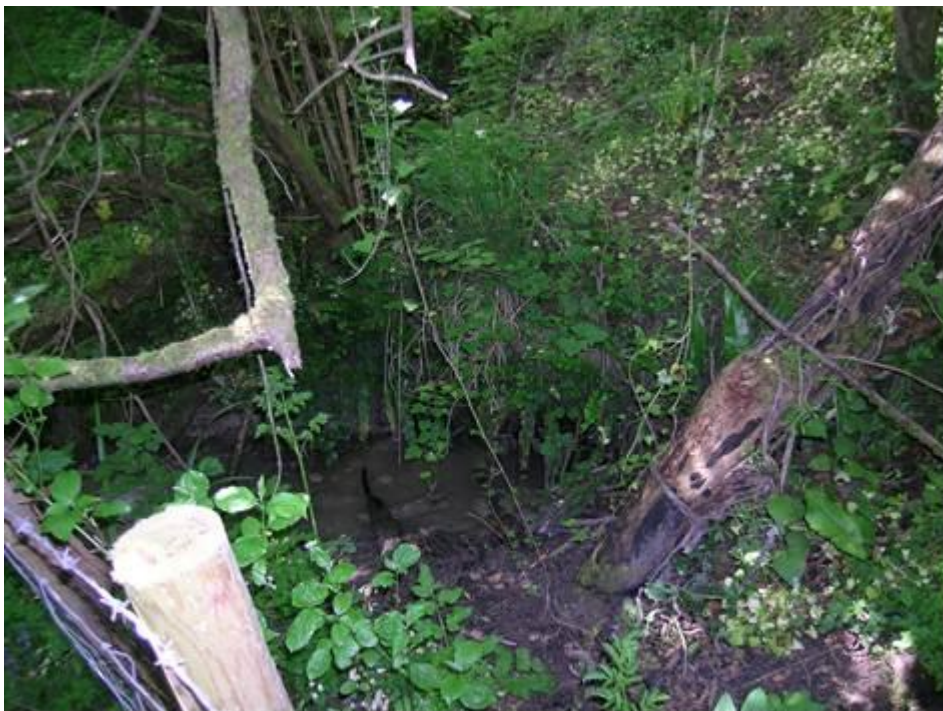
Figure 15. The fall from the impoundment into the culvert under the railway.
