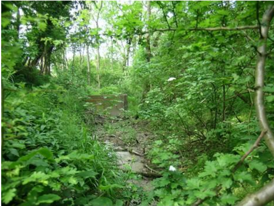
Figure 3. Concrete impounding structure on the eastern arm.
