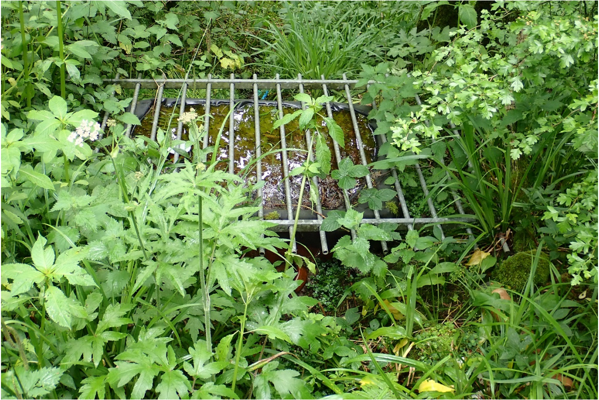
Possible private water supply, although use and ownership is not known.
