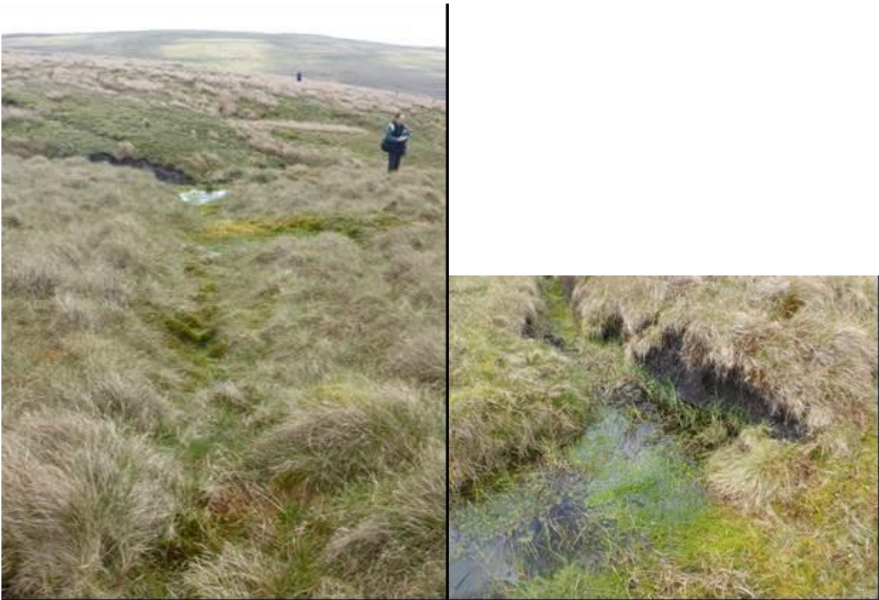
Figure 7. Path of former grip, now mostly filled in, and standing water habitat created by grip-blocking.
