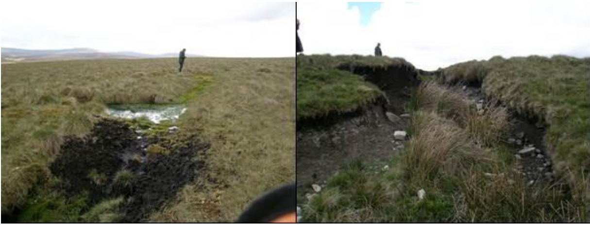
Figure 6. Gripping-blocking at the top of the ghyllside of Tyne Green Syke, showing the heavy erosion downstream of the peat plug prior to the connection with the stream.
