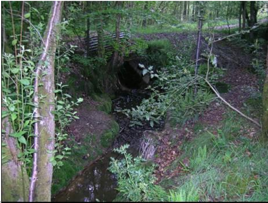
Figure 15. Culverting of Sheepwash Ghyll.
